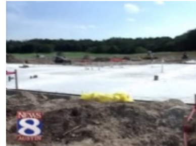
The foundation has already been laid for the new building.
